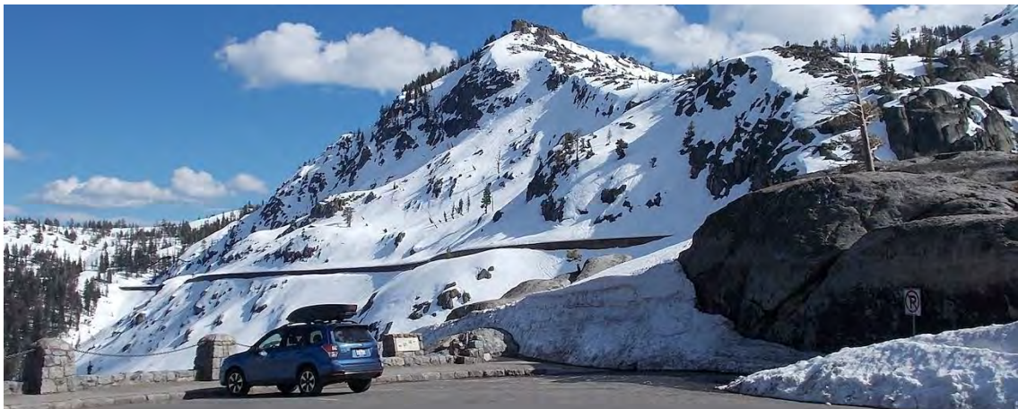
Railroad snowsheds cross the northeast face of Donner Peak, as seen from the Donner Pass Road vista point (DSCN6023.JPG).
