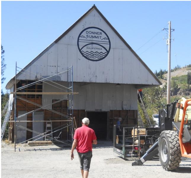
The Shed after completion of the logo painting task Friday afternoon. The forklift is at right. Scaffolding supports panel replacement on the east side, while a volunteer replaces lower roof fasteners using a ladder on the right (DSCN6445.jpg).
